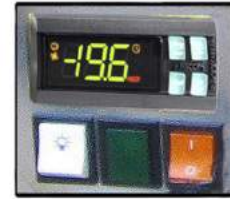
DIGITAL CONTROLLER WITH HIGH HEAD ALARM ON SELF CONTAINED
